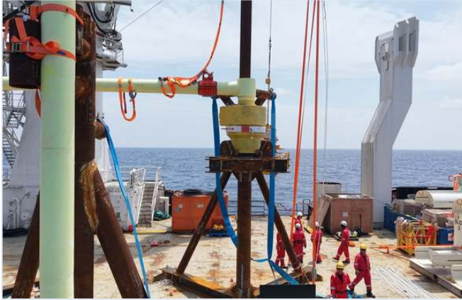
FIG 3.4-A — SOFT SLINGS CHOKED BENEATH SPREADER BAR
