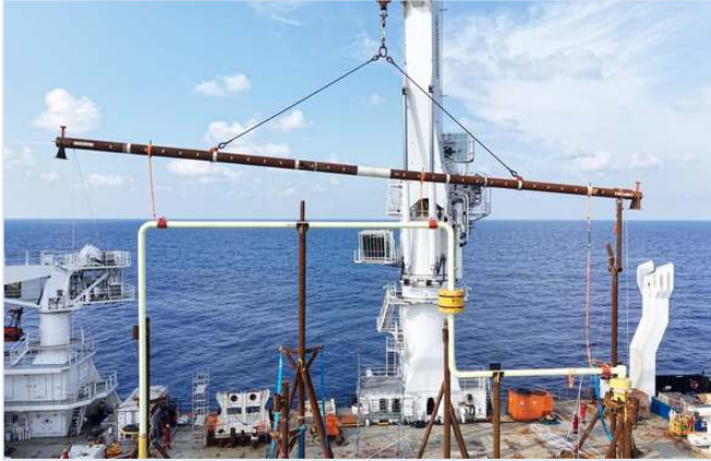
FIG 3.5-A — SPREADER BAR & CRADLE SUPPORT ARRANGEMENT
