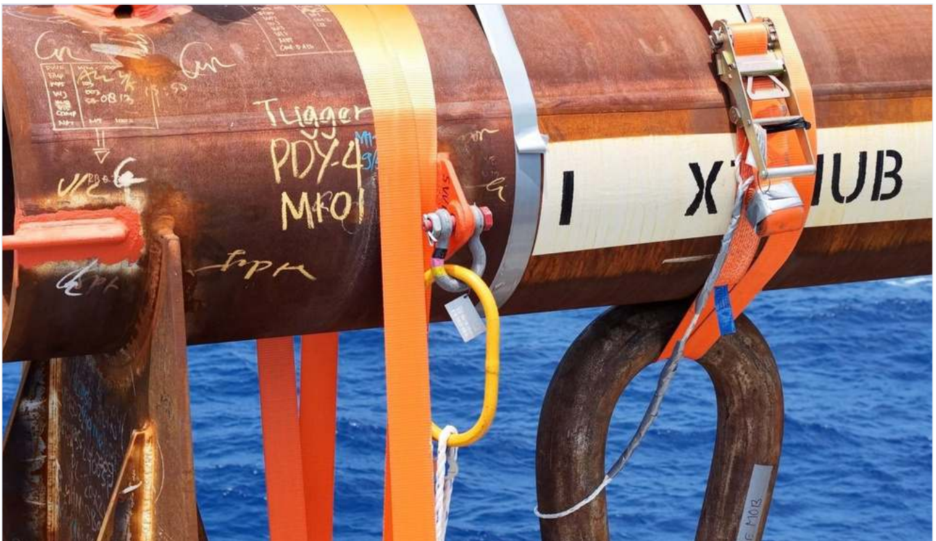
PLATE A-6 — CLUMP WEIGHT — RESTRAINT & CUT-AWAY RELEASE
