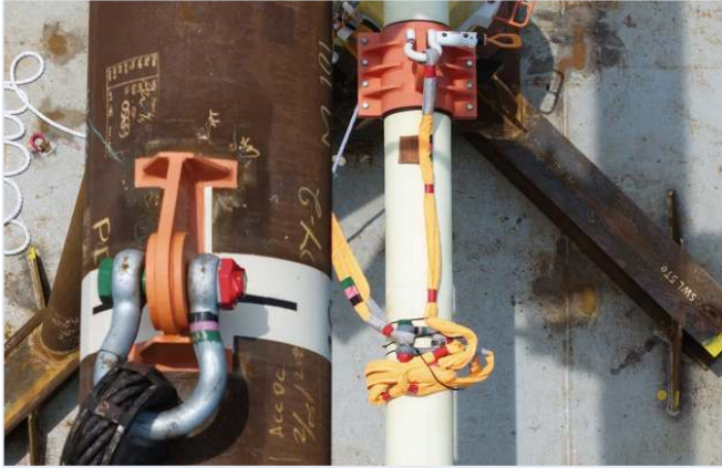
FIG 3.3-A — CHAIN LINKS & SPLIT PINS, TAPED AND SECURED
