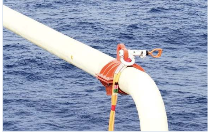
FIG 3.1-B — SHACKLE ORIENTATION & SLING EYE APPROACH
