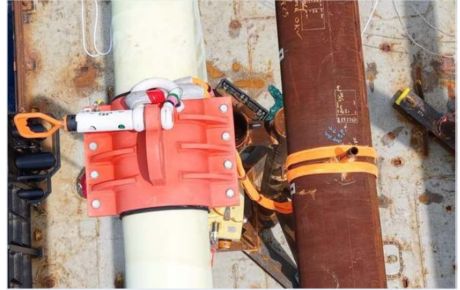
FIG 3.2-B — SLING EYE SEATED AT SHACKLE BOW TIP
