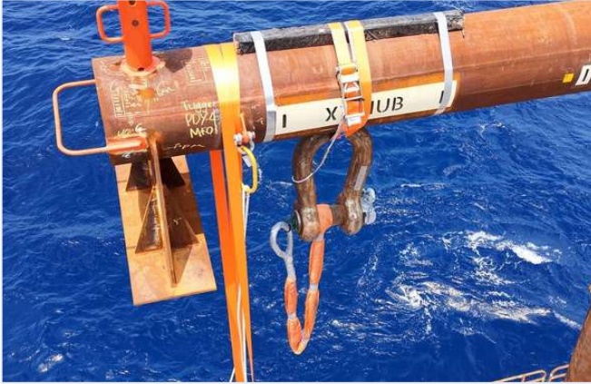
FIG 3.6-A — CLUMP WEIGHT SHACKLE RESTRAINT, CARGO STRAPS
